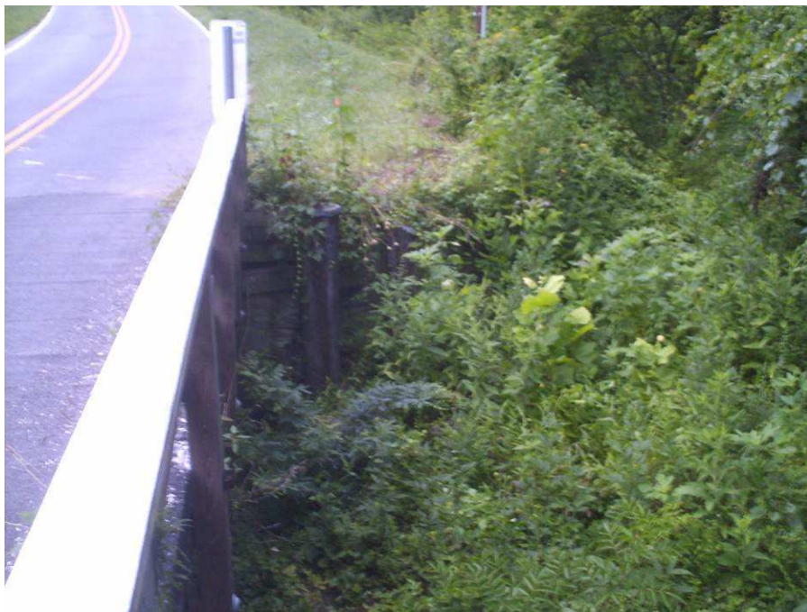
Photograph No. 8: View looking north at right side of End Bent 2
