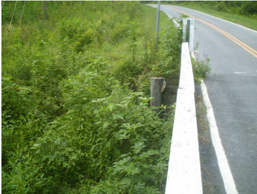
Photograph No. 7: View looking north at left side of End Bent 2
