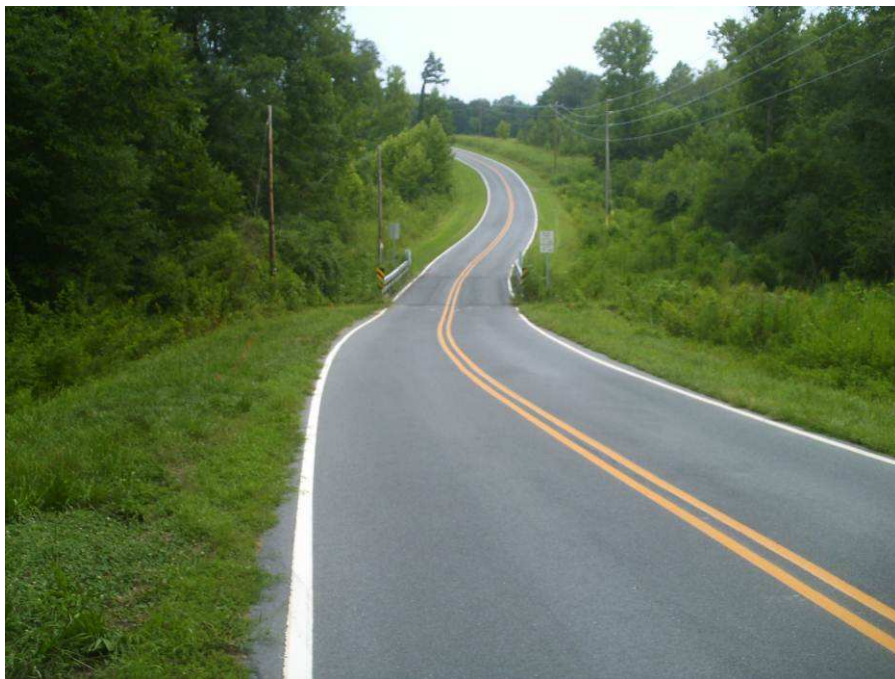
Photograph No. 2: View looking south down-station from north approach
