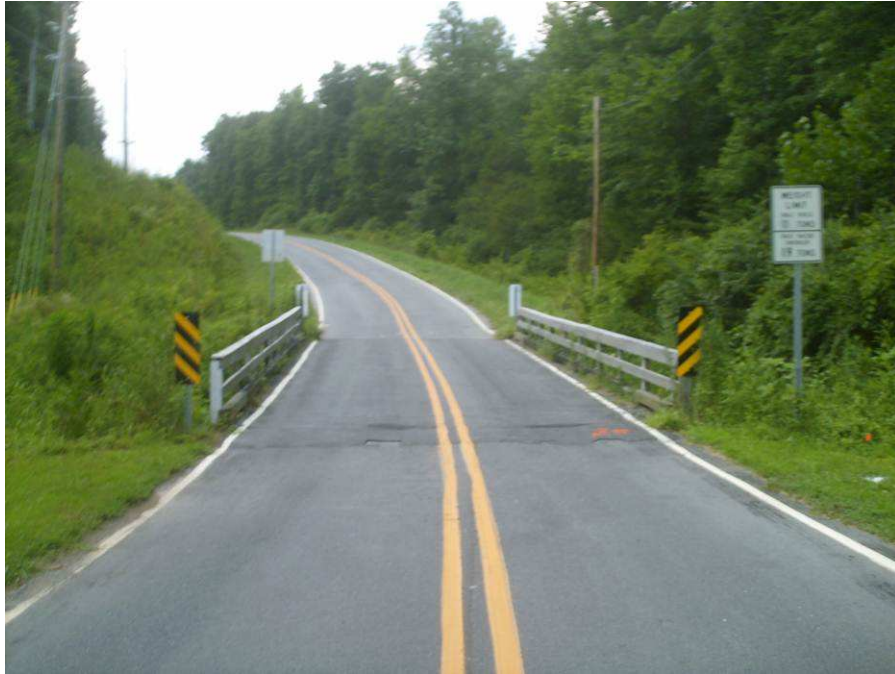
Photograph No. 1: View looking north up-station from south approach
