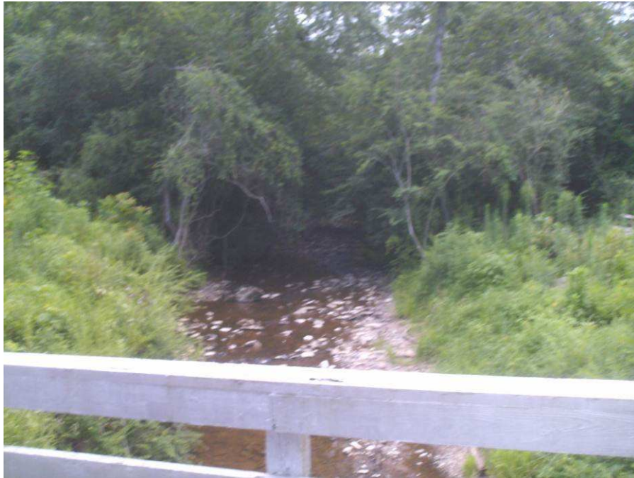
Photograph No. 3: View looking west upstream from bridge deck
