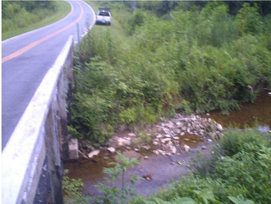
Photograph No. 5: View looking south at left side of End Bent 1
